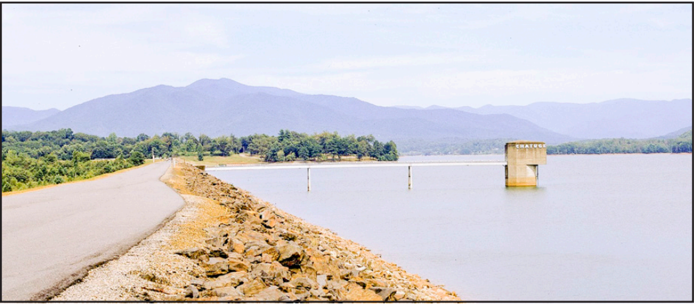
Chatuge Dam has been judged safe for normal operations in its current condition, but a vulnerability found in the spillway of the dam has prompted TVA to plan a fix that will begin construction in about three years. Photo/TVA.com
